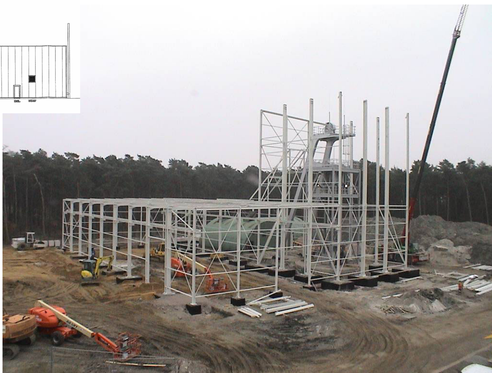
Figure 2: View of the lifting device of the main shaft and building site activities
