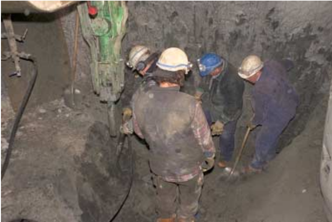
Figure 5-17: Second shaft: excavation in the frozen sands (jackhammer mounted on an hydraulic arm and manual air hammers).
