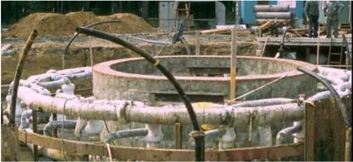
Figure 5-7: View of the top of the freezing tubes (approximately 250 m depth) around the location of the first shaft.
