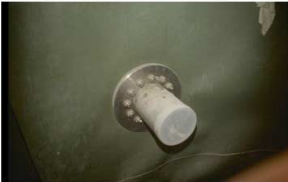
Figure 5-8: Passage of a measuring instrument through the watertight polythene membrane used in the lining of the first shaft.
