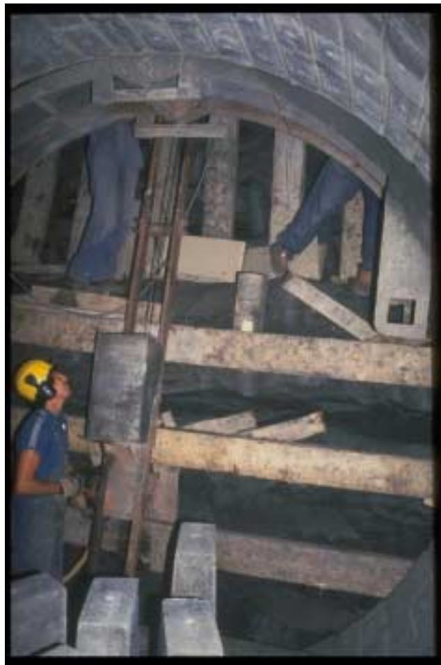
Figure 5-15: Test Drift: view of the lining made out of sliding steel ribs.
