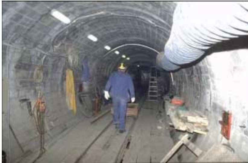
Figure 5-14: View of the excavation face of the Test Drift while emplacing the 60 cm thick concrete block lining.
