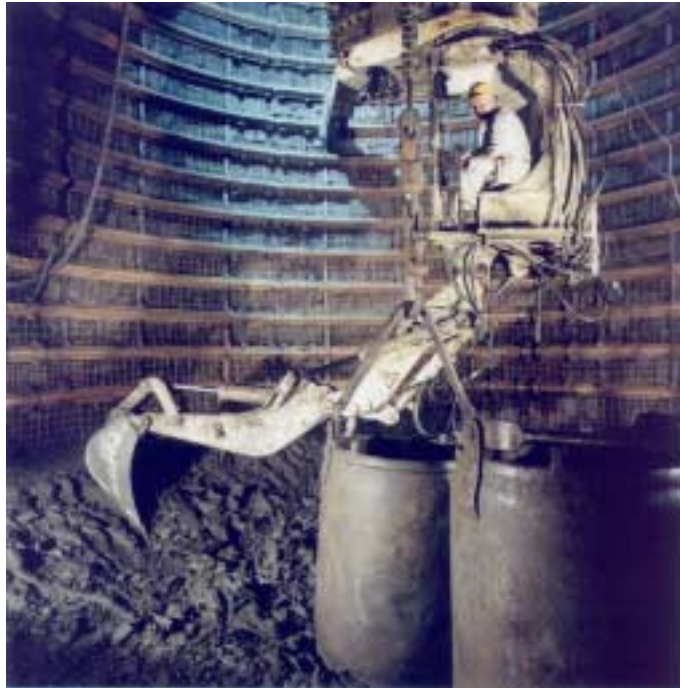
Figure 5-21: Second shaft: excavation method (hydraulic arm) and support (sliding ribs) below the foundation.
