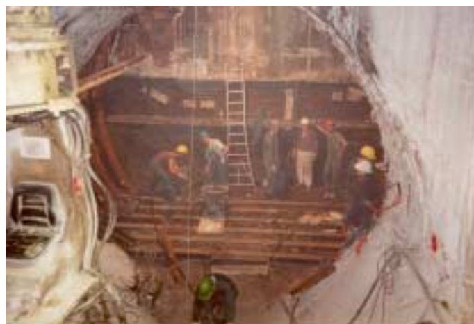
Figure 5-24: Second shaft: excavation of the starting chambers.
