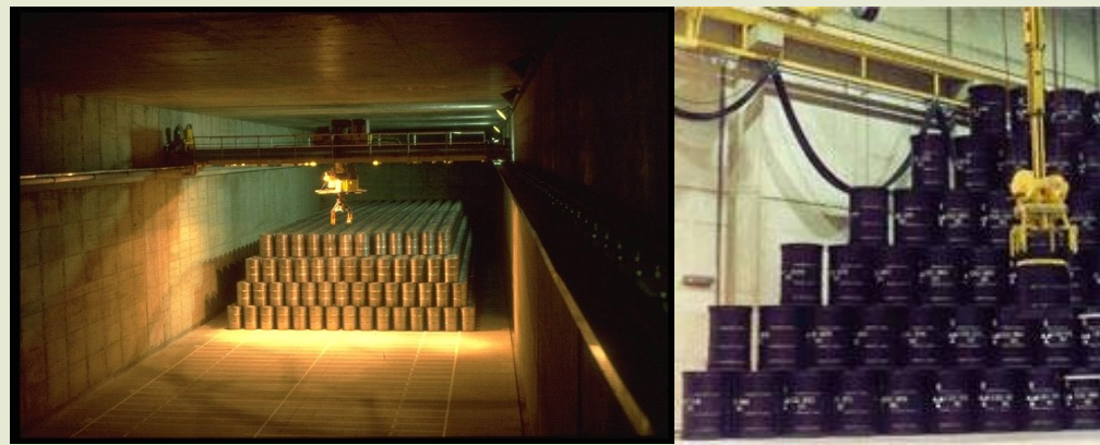
Figure 64 – Examples of interim storage of category B waste in Belgium. Left: The B127 interim storage facility contains bituminised waste. Right: The B151 interim storage facility contains low activity long life wastes (ONDRAF/NIRAS, 2008).
