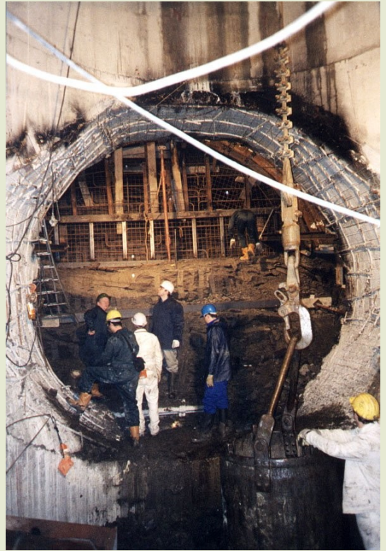
Constructing the chamber at the base of the second shaft
