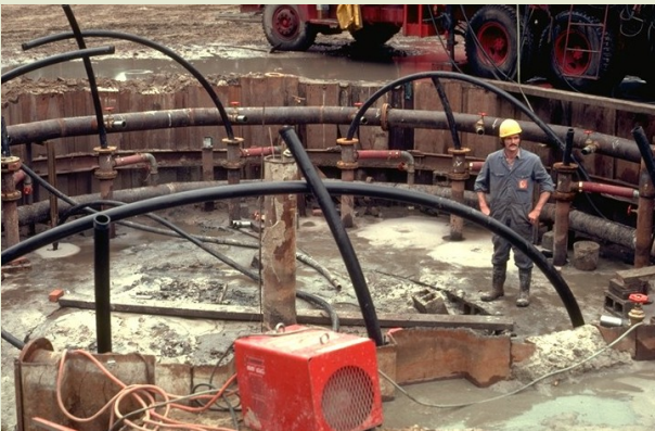
Freezing the soil with a view to constructing the first shaft
