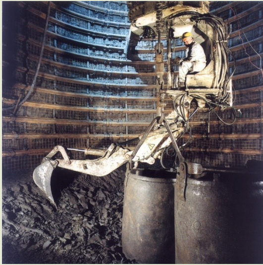
Constructing the second shaft
