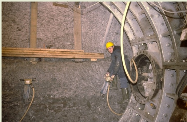
Excavating and fitting the lining of the first HADES URF gallery
