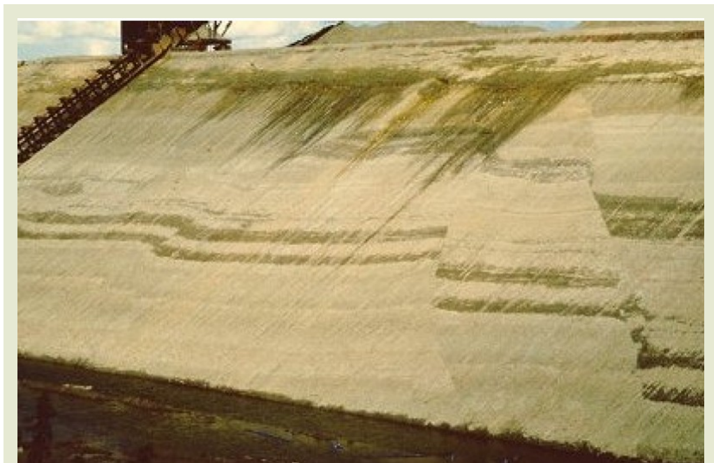
Figure 75 – Overview of a clay quarry (Marke) in the Ypresian clays, with potential onshore intraformational features as suggested by (Verschuren, 2001) (taken from ONDRAF/NIRAS, 2001).
