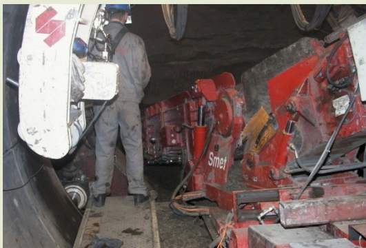
Constructing the Connecting gallery using a tunnel boring machine
